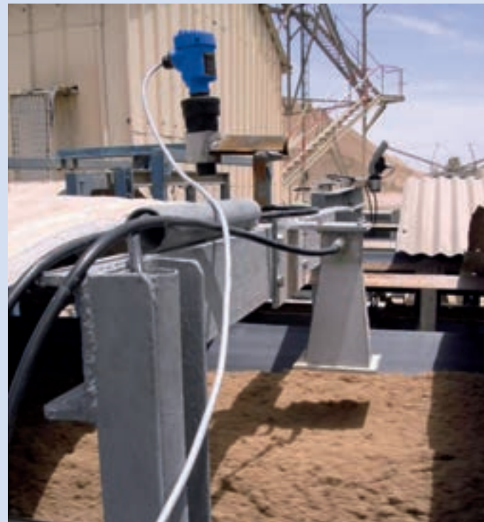
Moisture measurement of phosphate - LB 567 with horn antennas in combination with an ultrasonic height sensor in order to compensate for the varying bulk material heights.
